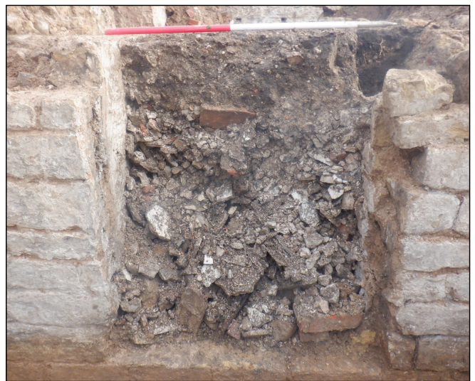
Plate 14: Doorway into Cellar 2, looking east
