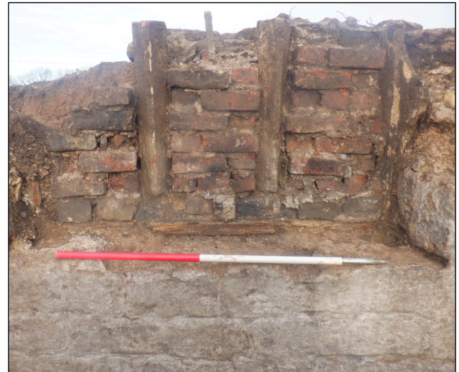
Plate 11: Window 13042, looking north
