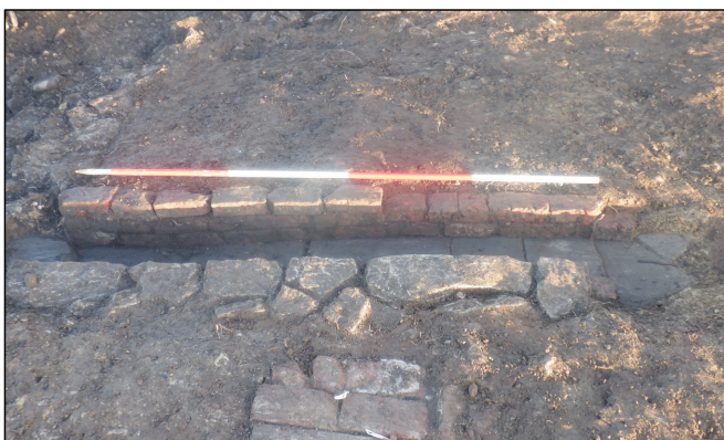
Plate 21: Culvert 13015, looking south
