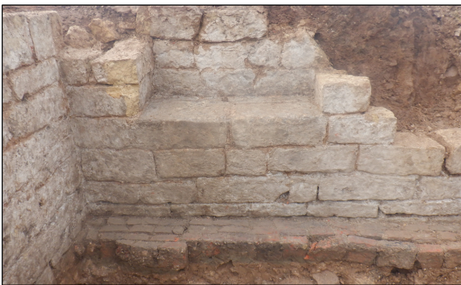
Plate 13: Elevation of the cellar wall showing a brick floor at the base, looking north-west
